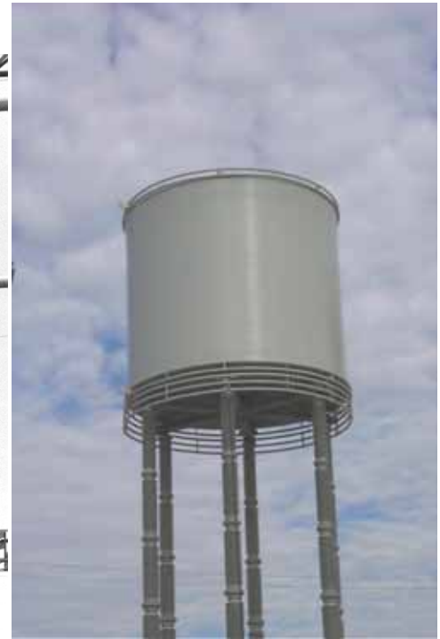
New style air-cored smoothing reactor
