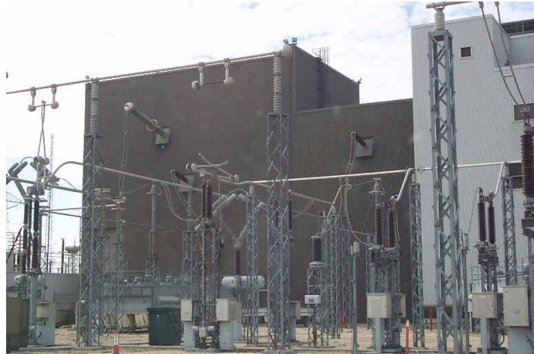
Top: DC Side Bushing in Valve Hall
