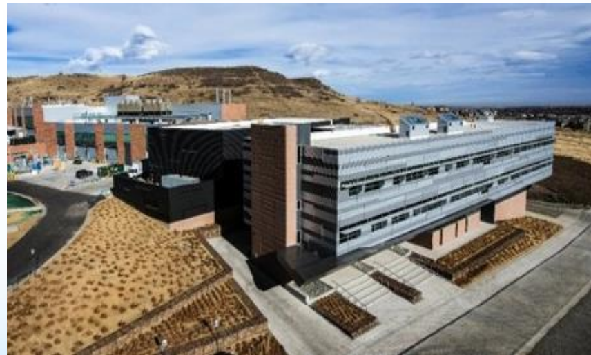
Energy Systems Integration Facility (ESIF)
